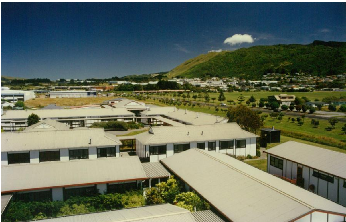
Aerial view of the Porirua campus and the health block comprised of prefabs surrounding interior courtyards
