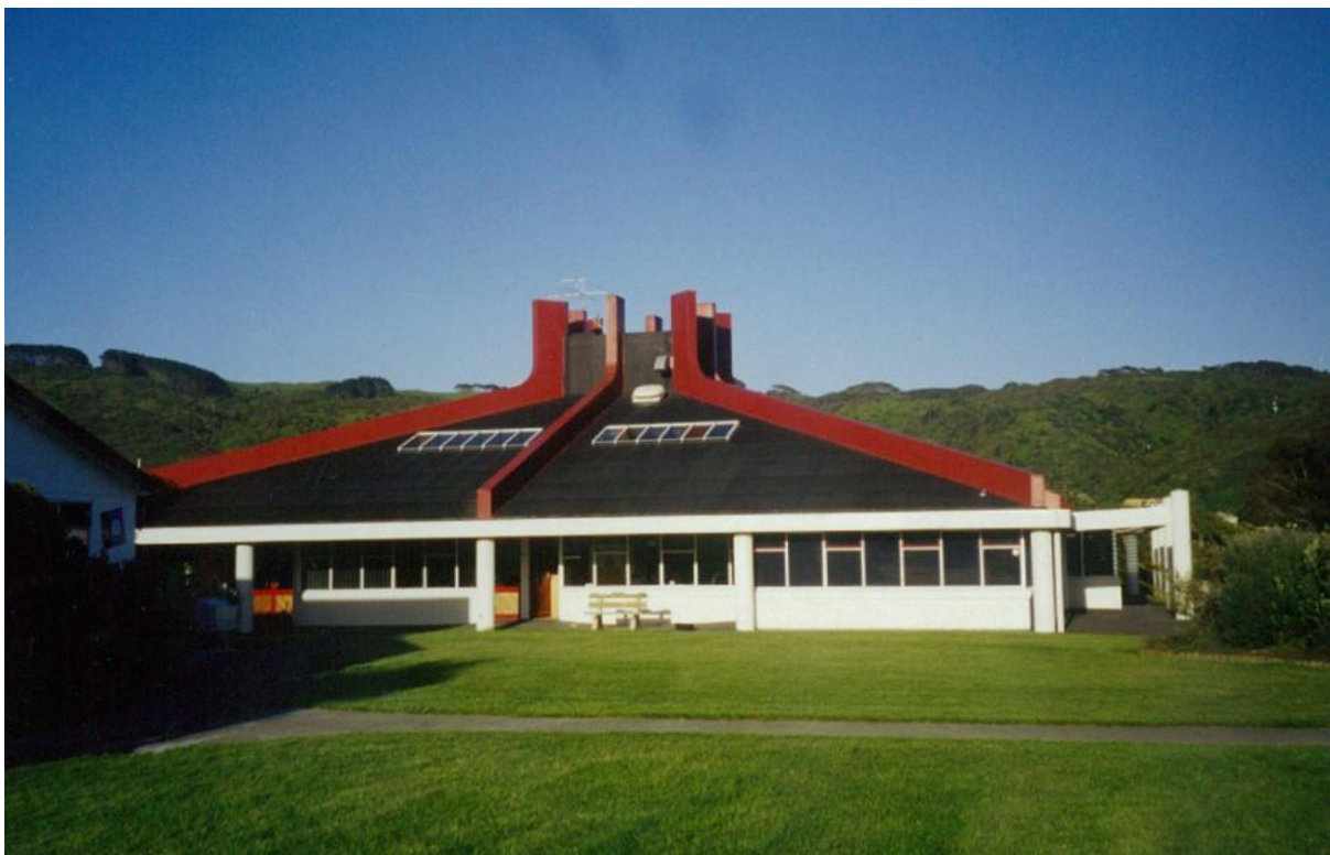
The wing of the Administration Building at Porirua campus named after Governor-General Sir Paul Reeves
