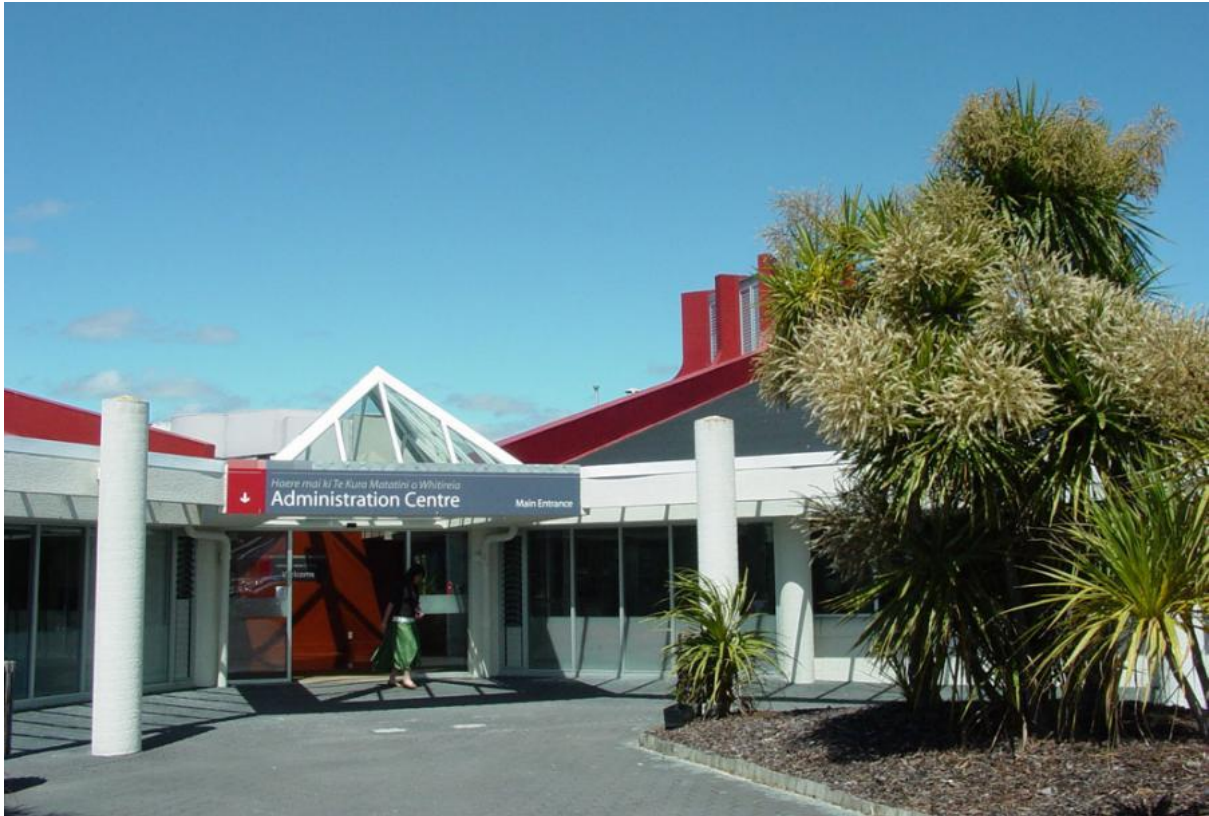
Entrance to the administration building in 2002
